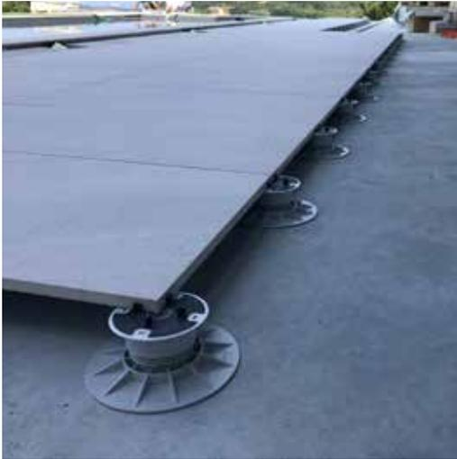
For this elegant outdoor and poolside area of a private villa in Slovenia, the solutions of the DPS Solving collection were chosen to **create one multilevel raised flooring**, which would allow comfortable and safe access to the pool floor and at the same time the invisibility of the systems under the flooring, which can always be inspected.
