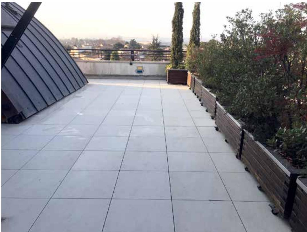
**The renewal of the paving of a large terrace located on the top floor of an apartment building in Spresiano (TV)** was necessary due to serious infiltrations caused by damaged waterproofing.
